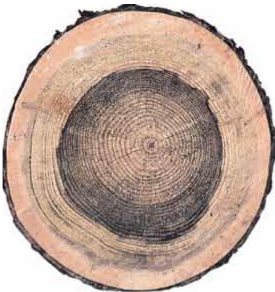
A clear, dark zone marks the boundary between the rot in the middle of the disc and the aniline wood. The entire dark area is assessed as dark rot. If the rot continues to develop, it first becomes soft rot and finally forms a rot hole.
